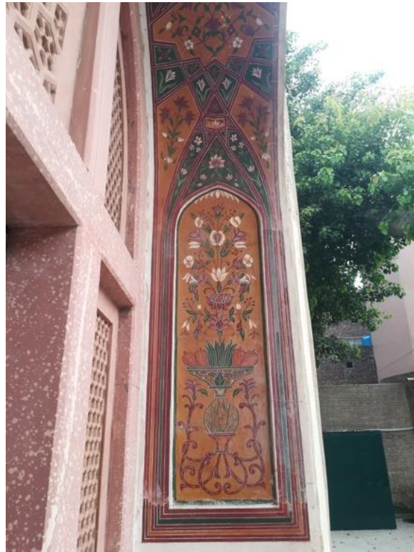
Fig 29: Paint work on arch of Tomb
