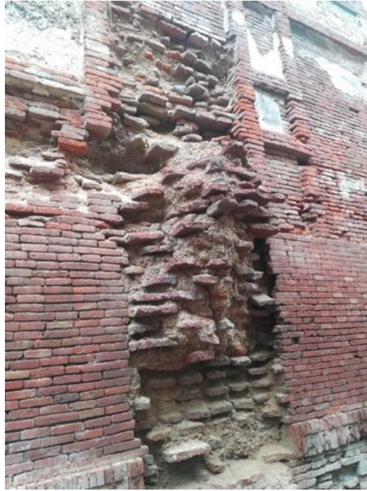
Fig 24: External wall of Chauburji
