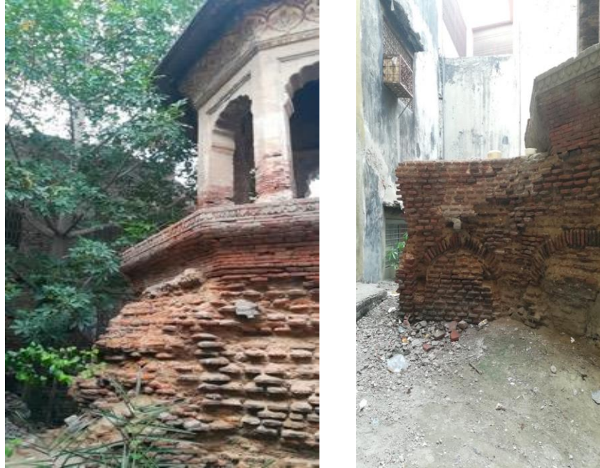
Fig 15: External wall Burj 1 and 2
