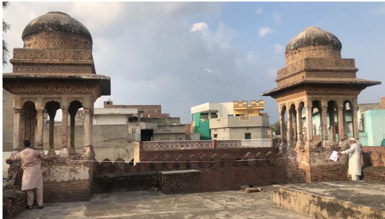
Fig 23: Measuring Roof of Chauburji
