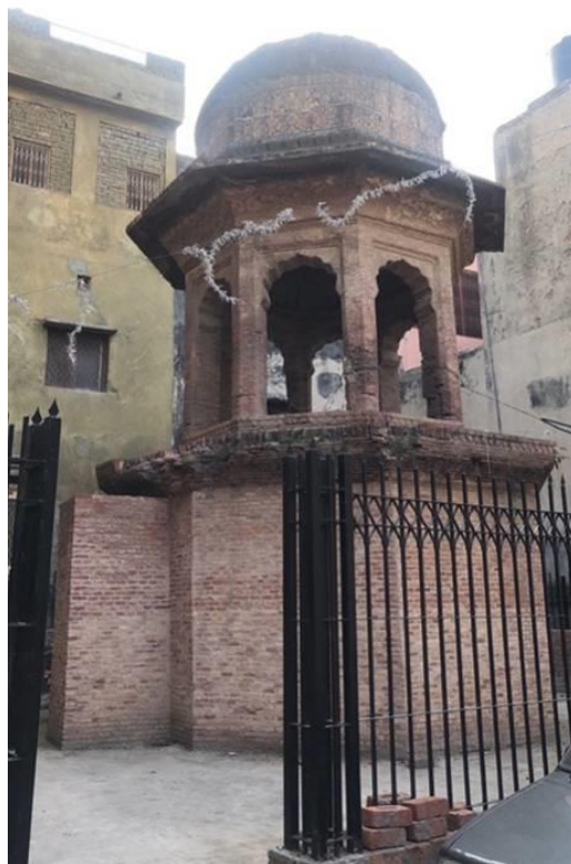
Fig 37: Iron gate at Burj 2
